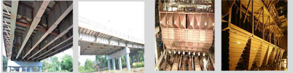
Road over bridge at Behrampore, Kishangarh
