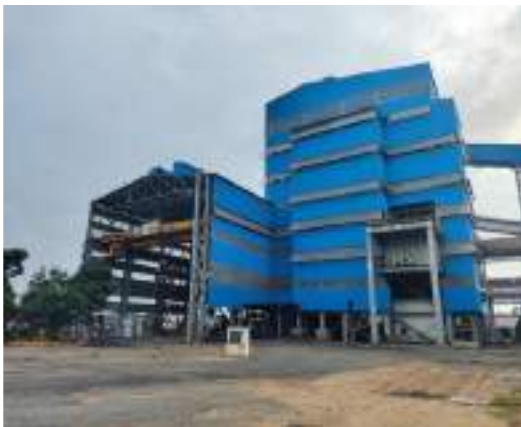
FURNACE BUILDING AND CAST BAY
