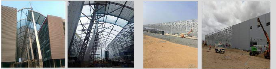
Canopy Structure at TCSHyderabad
