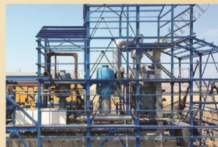
Solvent Extraction Plant
