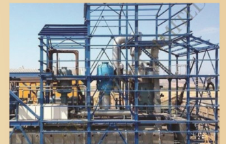
Solvent Extraction Plant
